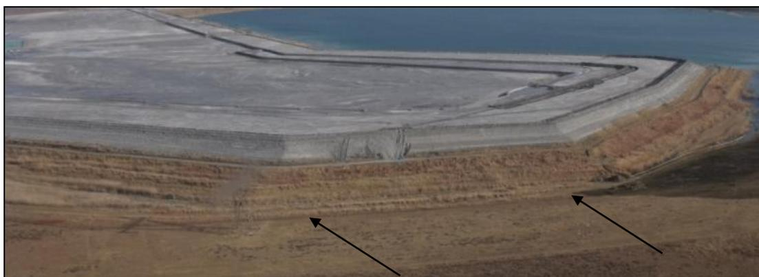
**Figure 7-11: Rehabilitation on the existing ash disposal site in the foreground**
